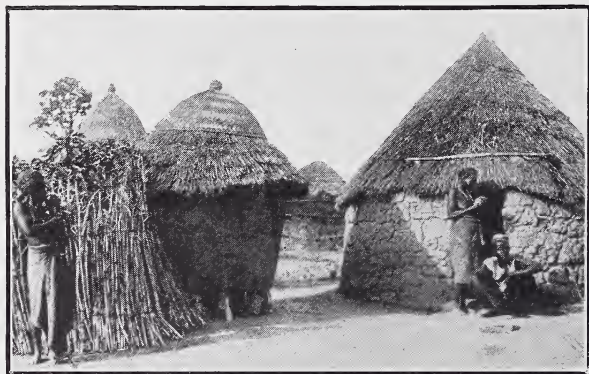
Round huts with mud walls and thatched roofs common in the southern districts of the Cameroons.
